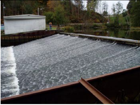
Metal dam constructed of sheet pile
