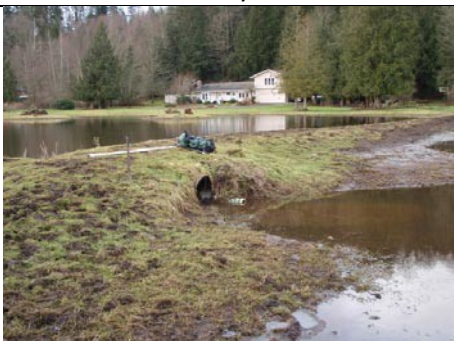
Earthen fill dam
