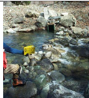
Rock fill dam and diversion
