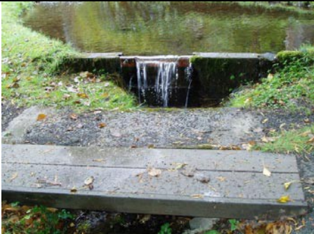
Full span concrete dam with removable wooden boards
