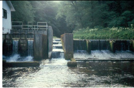
A concrete dam with a weir-pool fishway
