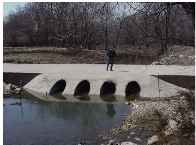
Figure 14. This low water crossing has larger vents that were set well below the channel elevation. This might be acceptable where there is little danger of channel incision for the life of the structure.
