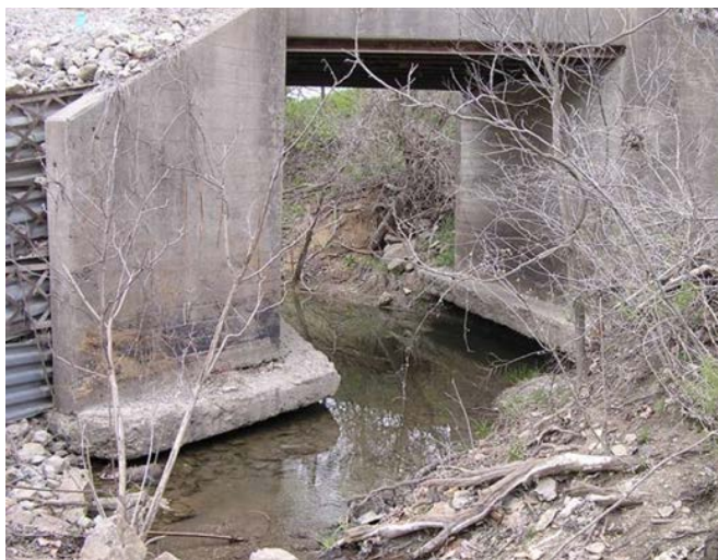
Figure 9. Channel incision has exposed the bridge footings.
